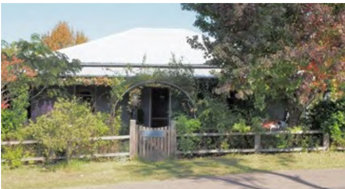
Dating from 1823, Longleat Farm in Longleat Lane gave its name to the area which is now called Kurmond. The house was originally built in 1865 and was surrounded by orange orchards. It was the home of the Chapman family in the 1930s. In the last twenty years it has been restored with sympathetic additions by Colin and Ros Tomlinson. Ros has created a beautiful cottage garden. (K-CHS LEP Item: 458)
