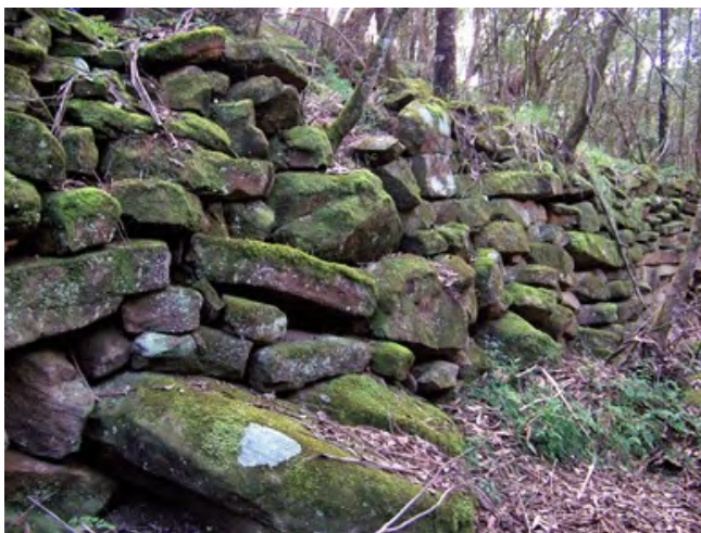
MILL RACE WALL - Lower Mill Site Wheeny Creek
