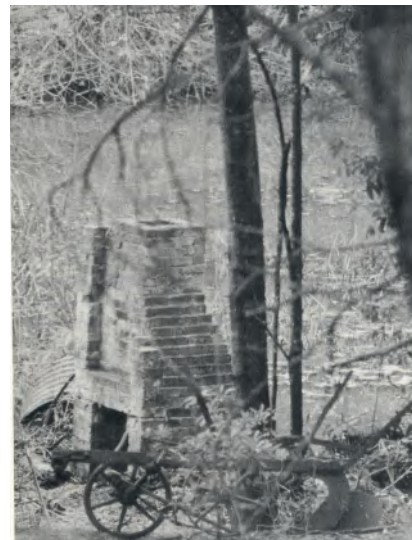
Chimney & remnant farming equipment Mackenzie home, Hermitage Road, Kurrajong
